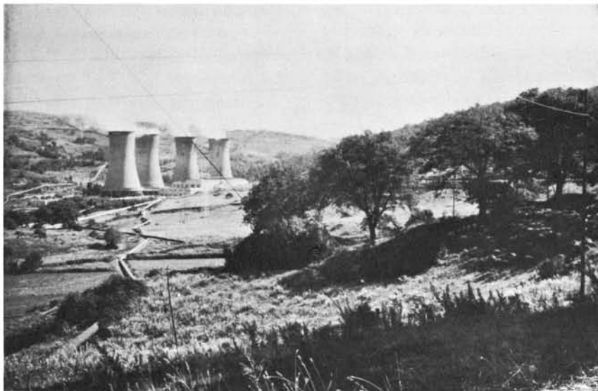
Figure 5. Larderello power plant with steam-gathering lines passing through an orchard in the foreground. This site has been used for electric power generation for over 60 years with only minimal environmental impact. (Photo by Ira E. Klein, U.S. Bureau of Reclamation)
